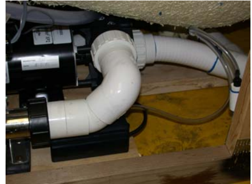
Completed Ozone connections. Figure 26
