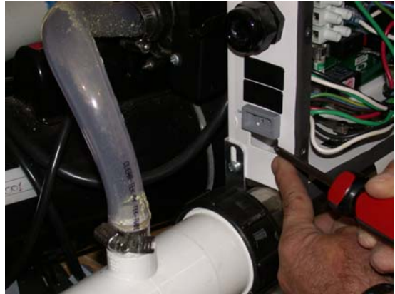
Remove Circ. Pump/Aux hole cover Figure 5
