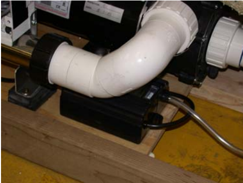
Connect ozone tube to CD unit. Figure 25
