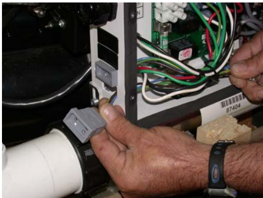
Install J&J connector Figure 6
